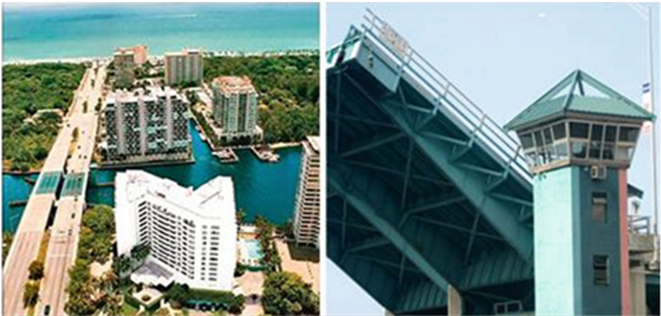
Fig. 42.2 Sunrise Boulevard Bridge (SBB)
