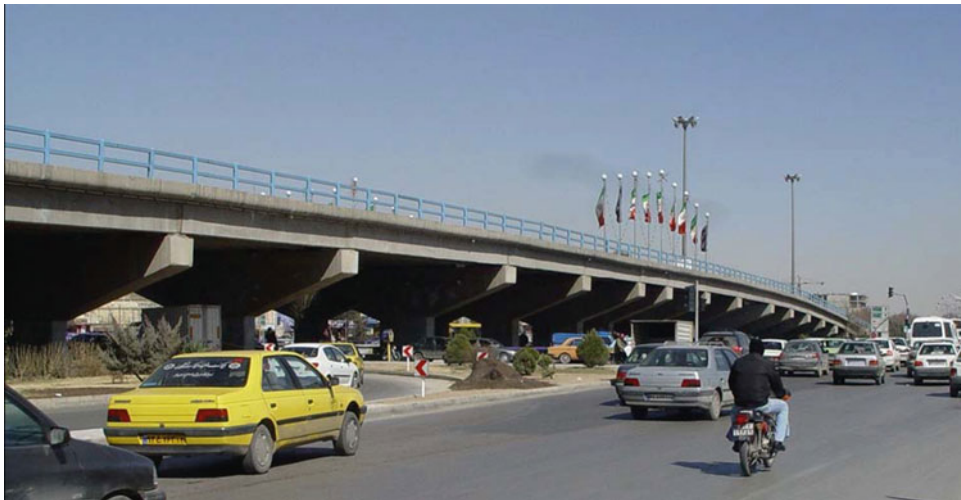
Fig. 18.2 Bridge elevation and vehicle traffic below
