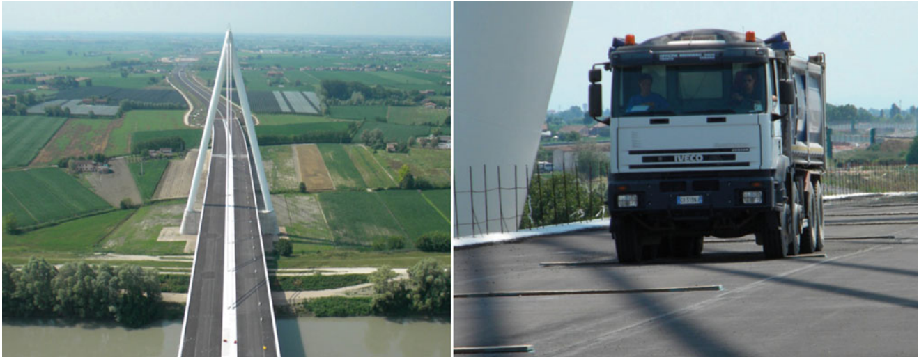
Fig. 17.2 Aerial view on the bridge and truck passing on the obstacles on the deck
