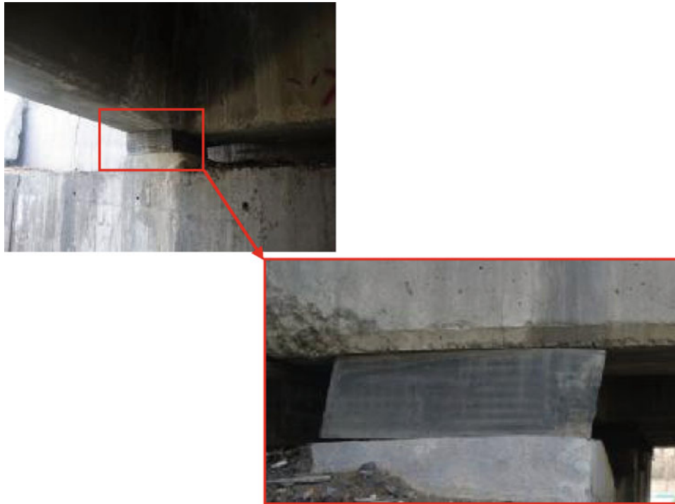
Fig. 18.7 Local damage in isolators
